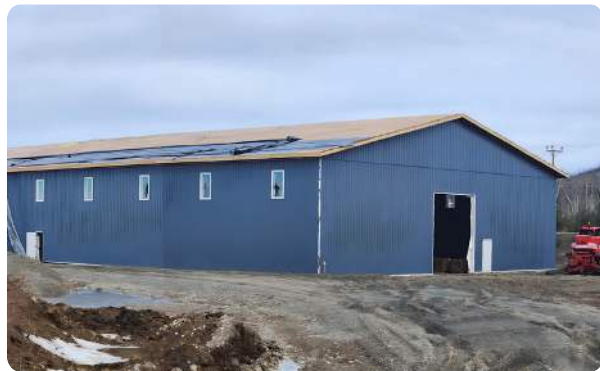
Construction of the Healing and Wellness Center.
