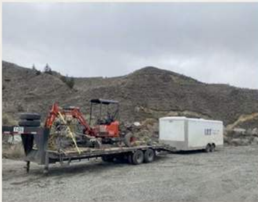
Axis equipment mobilized to left bank.
