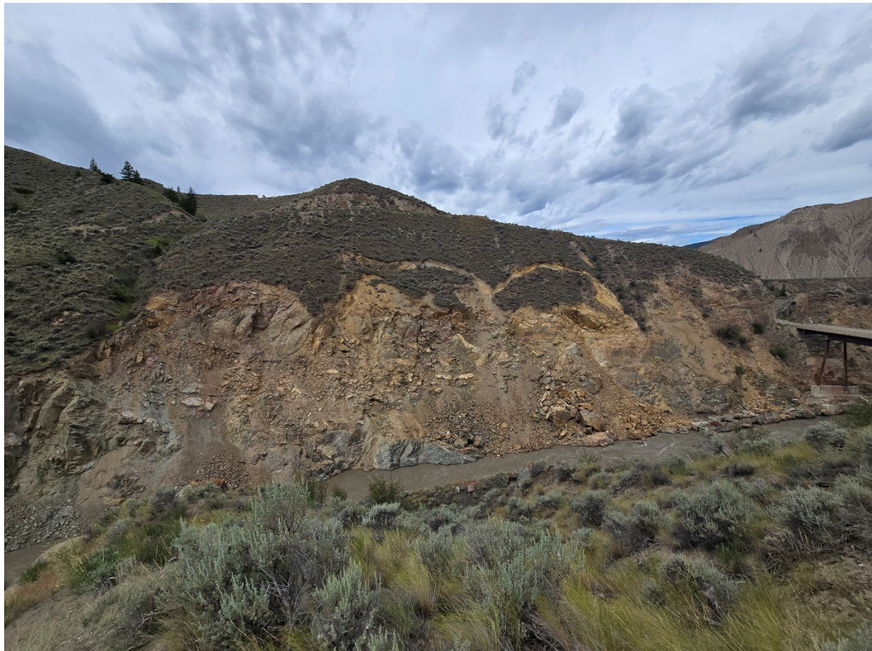
Figure 11 Overview photo of the Farwell Canyon slope tension crack that resulted from 2024 breakout flood, taken on July 02, 2025.
