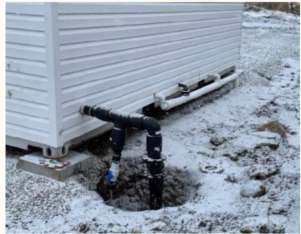
Water hook-up for the TNG interim hatchery, connected on February 15, 2023.
