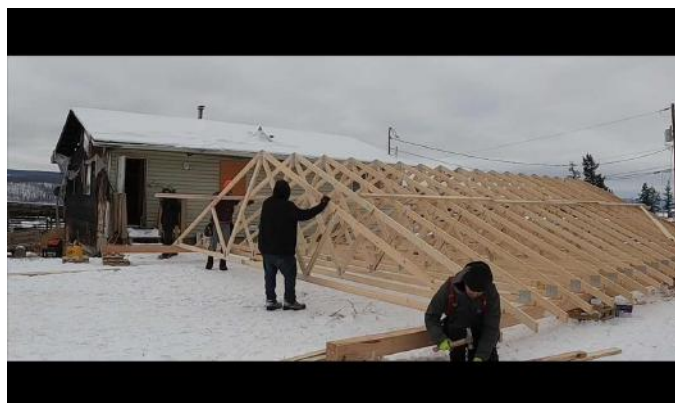
[PHOTO 1] Caitlin putting up a roof in Tl'etinqox.
