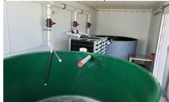
Caption: Standard Hatchery-in-a-Box c-can interior with rearing tank and incubation trays.
