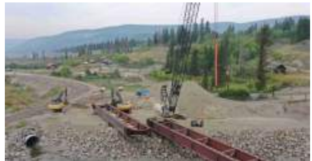
Photos of the girder launch that was recently done on the Zenzako bridge
