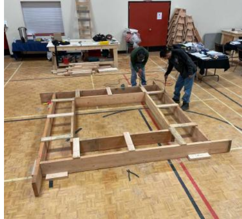
Photo 1: Footing Formwork
