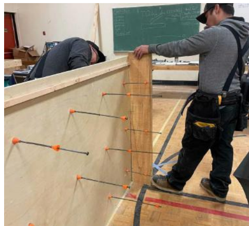
Photo 3: Forming Bulkhead
