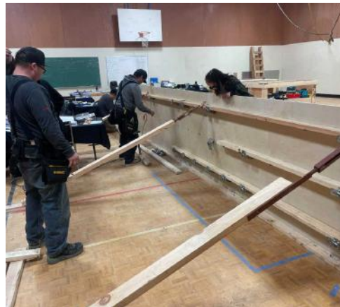
Photo 2: Footing Bracing
