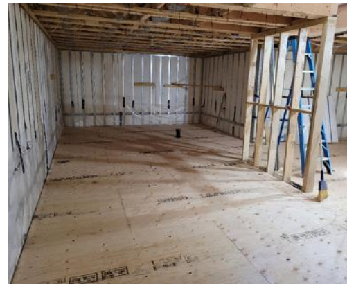
Photo 2: Styrofoam and steel wall system that replaces concrete
