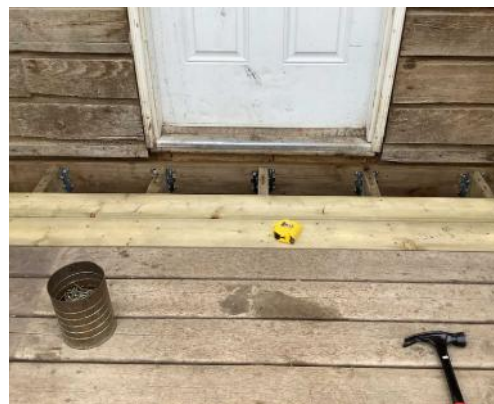
Photo 1: Decking in Tl'etinqox
