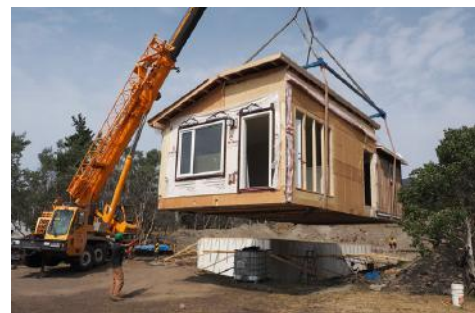
Photo 1: House in place.
