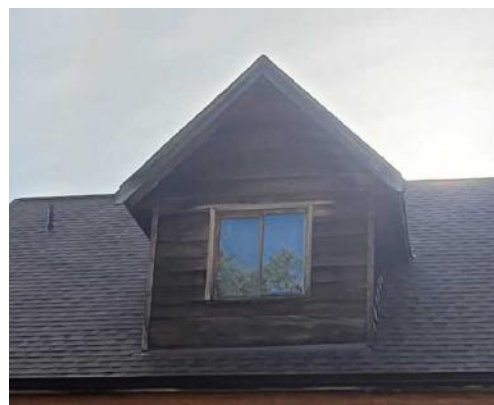
Photo 1: Roofing for Tl'etinqox
