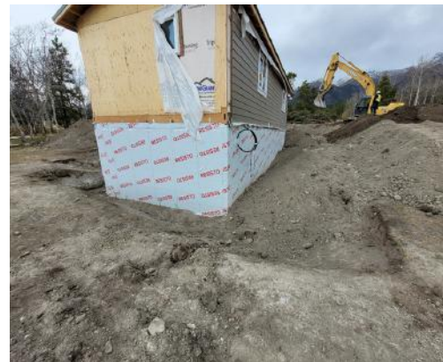
Photo 3: Backfill starting on a foundation in Xeni
