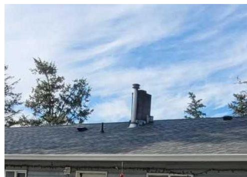
Photo 2: Gutter work in Tl'etinqox.
