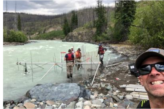
Photo 4: TNG Fisheries Biologist Pete Nicklin and the TNG and DFO crew installing the Taseko SONAR system to count sockeye and chinook migrating through the Taseko River.
