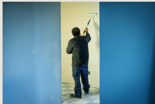
Renovations being done in Tl'etinqox
