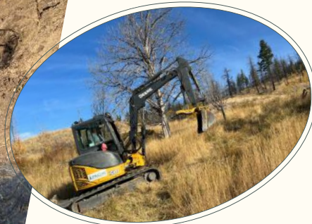
Preparing the hatchery site at Hanceville for hatchery installation
