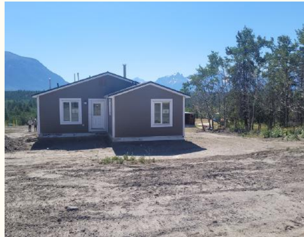
Completed RTM home in Xeni Gwet'in
