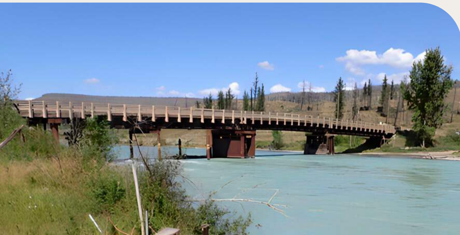
Hanceville Creek and Henry Bridge
