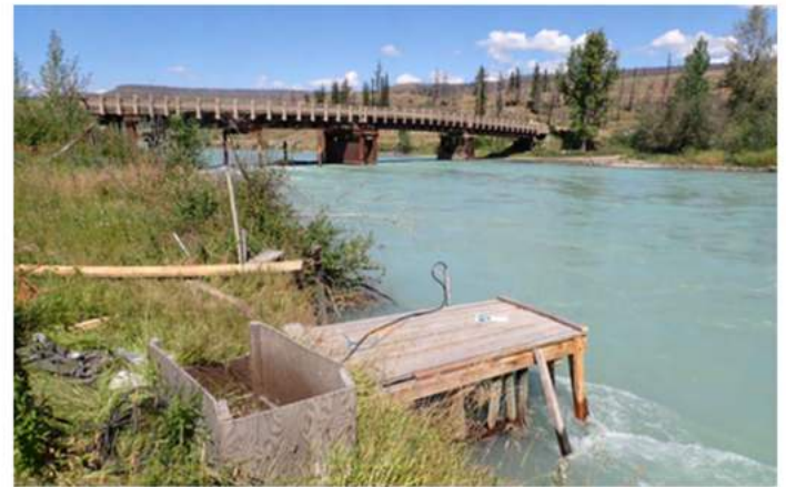
Photo of station installed on the Chilcotin River near Farwell Bridge (Aug 14)
