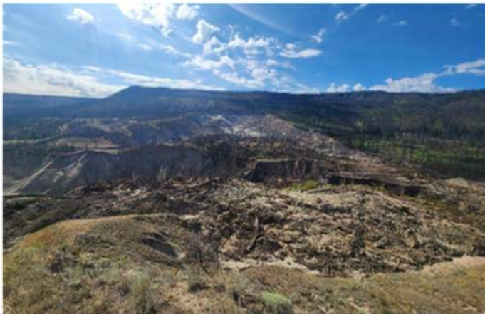
Photo of slide area looking south (Aug 14-15)
