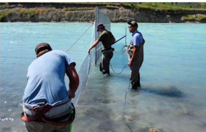
TNG Fisheries crew worked with technical partners from EcoFish Research Ltd. to install a new fish passage SONAR upstream of the slide at Hanceville on (Aug 8)
