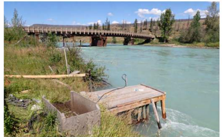
Photo of station installed on the Chilcotin River near Farwell Bridge (Aug 14)
